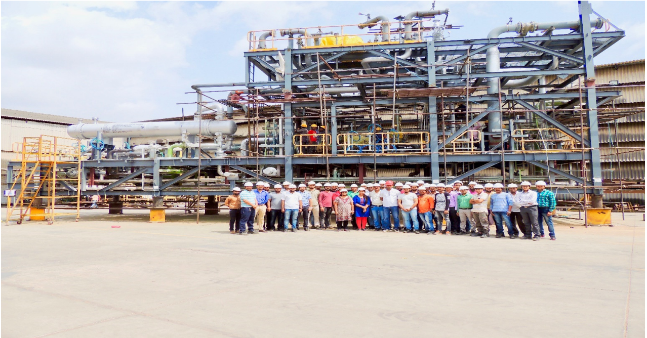
Cryogenic Hydrogen Recovery Unit (CHRU) Client: - Linde Engineering India Pvt. Ltd. End User:- Ramagundam Fertilizers & Chemicals Limited (RFCL) Telangana
